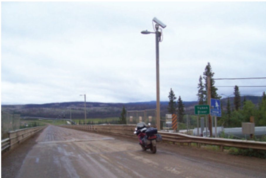
The bridge at Yukon Crossing is decked with planks, now wet and slippery.
